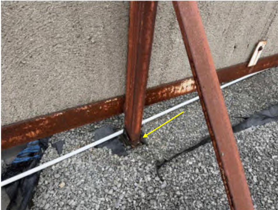
Photo #17: Example of Pitch Pocket at Pre-cast Concrete Screen Structural Steel Support – IRMA Section. Steel has Corrosion at Base
