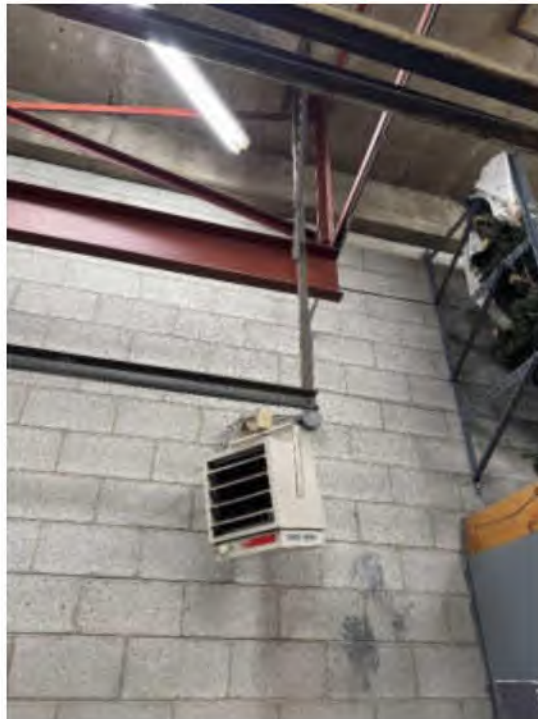
Photo #26: Loading Dock Electric Unit Heater
