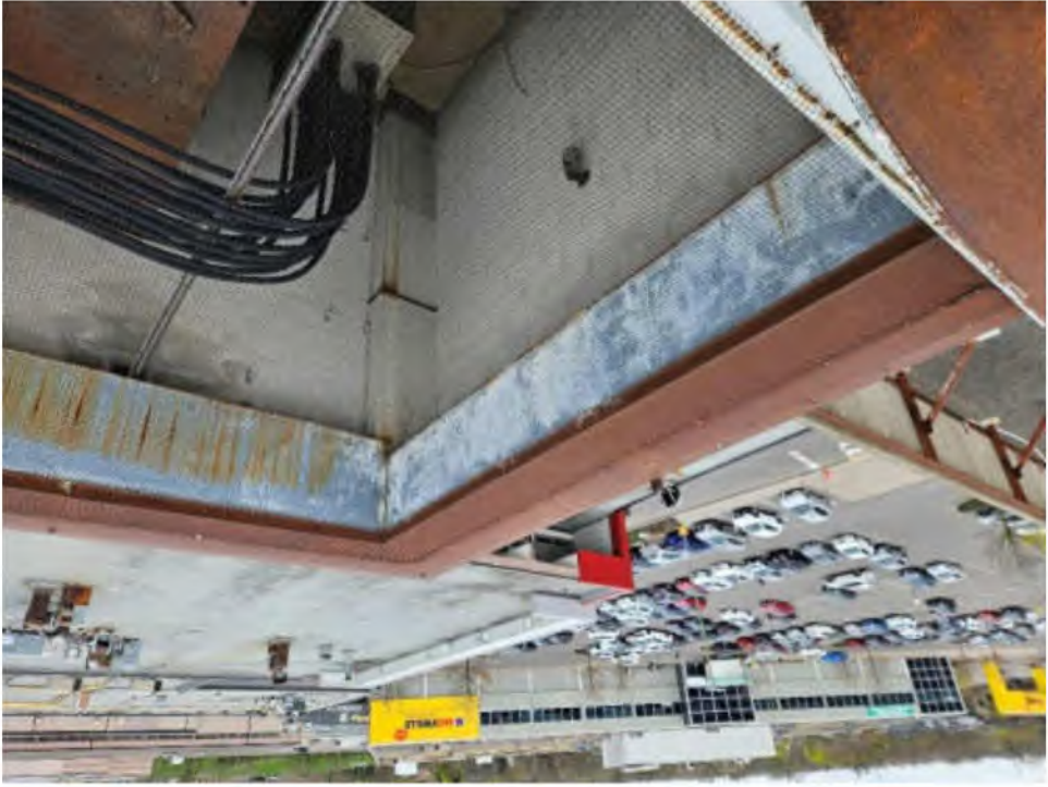
Photo #11: Example of Corroded Cap Flashing (Mechanical Area)
