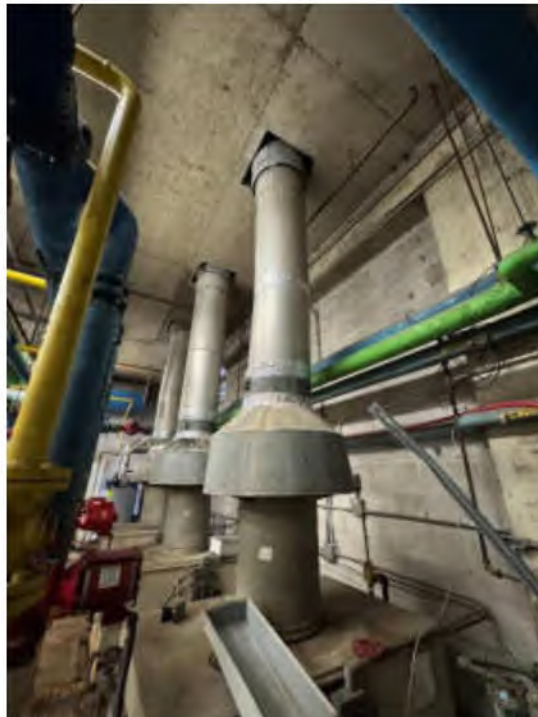
Photo #10: Heating Boilers Venting System
