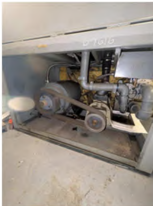
Photo #10: Freight Elevator Power Unit Pump
