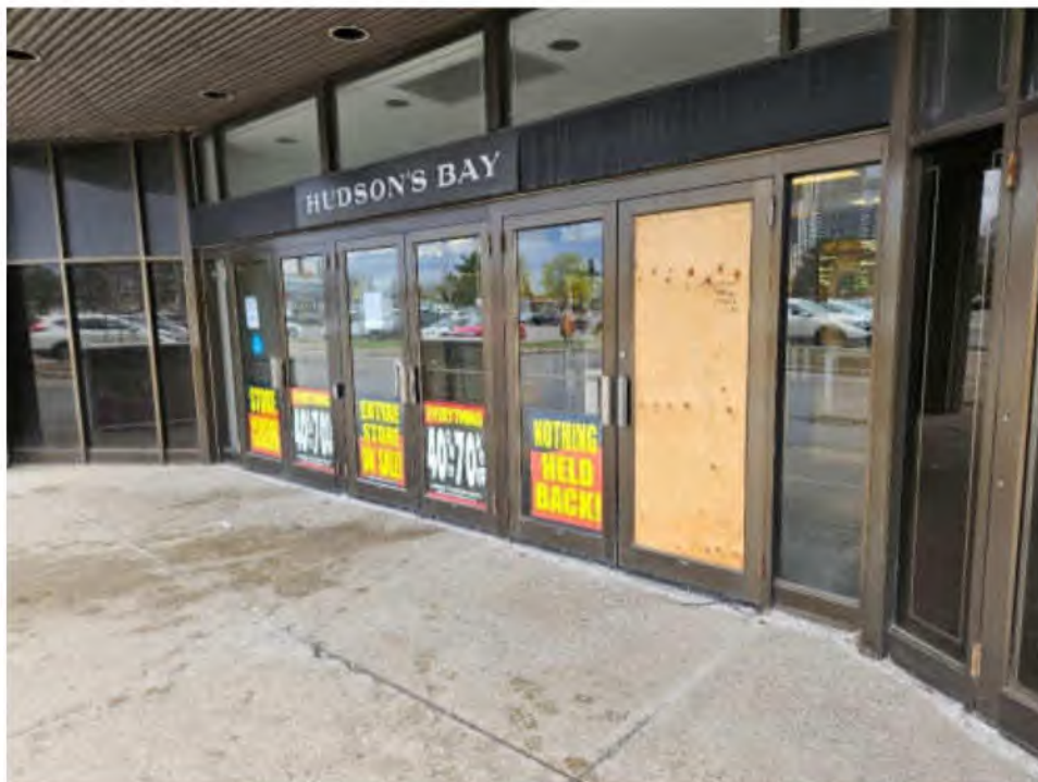
Photo #30: Damaged Storefront Window Glazing
