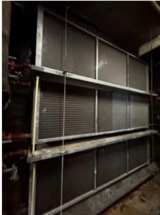
Photo #13: AHU-1 Dual Temperature Heating/Cooling Coil
