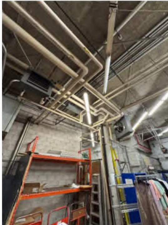
Photo #21: Loading Dock Hydronic Unit Heaters
