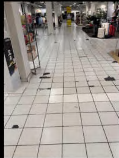
Interior - Duct tape over damaged floor tiles, water leaks, carpet condition
