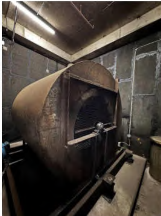
Photo #12: First Floor Air Handling Unit Supply Fan (AHU-1)
