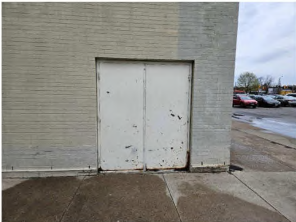
Photo #32: Example of Corrosion at Service Doors
