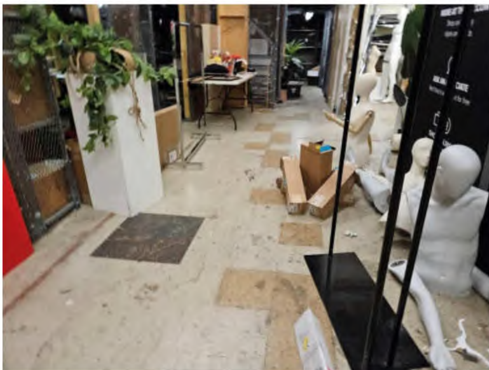
Photo #13: Example of Vinyl Tile Condition
