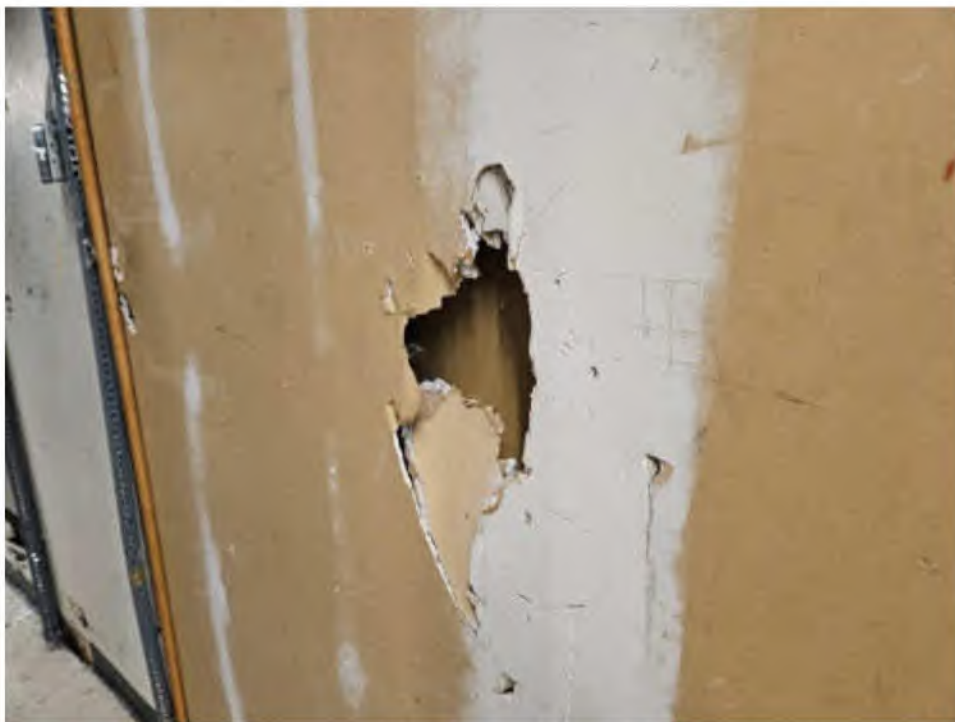
Photo #14: Example of Damaged Gypsum Board at Service Areas
