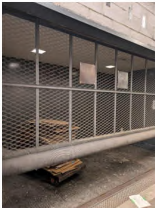
Photo #6: Freight Elevator Car Gate
