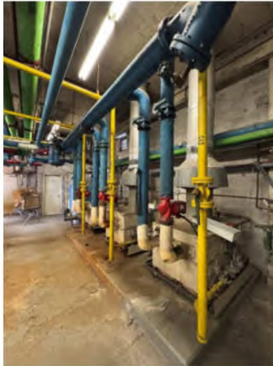
Photo #7: Gas Fired Heating Boilers
