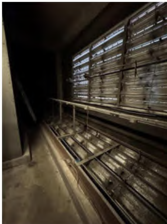
Photo #16: AHU-2 Mixing Air Plenum
