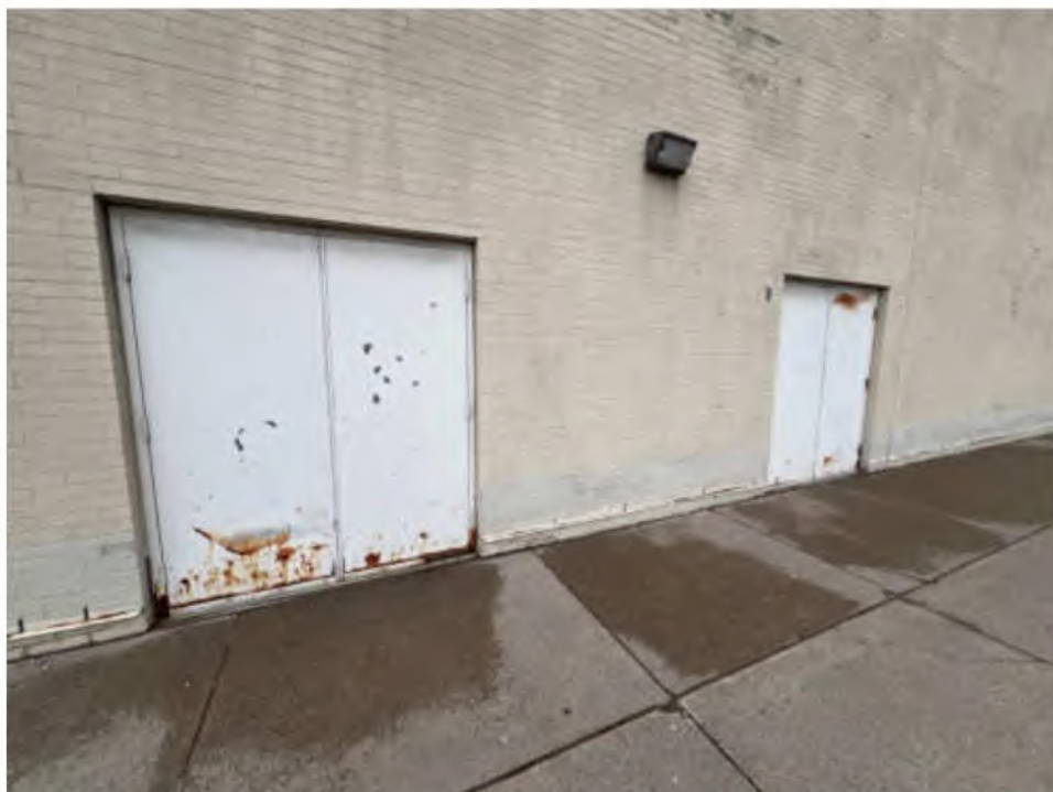
Photo #10: Typical Hollow Metal Service Doors
