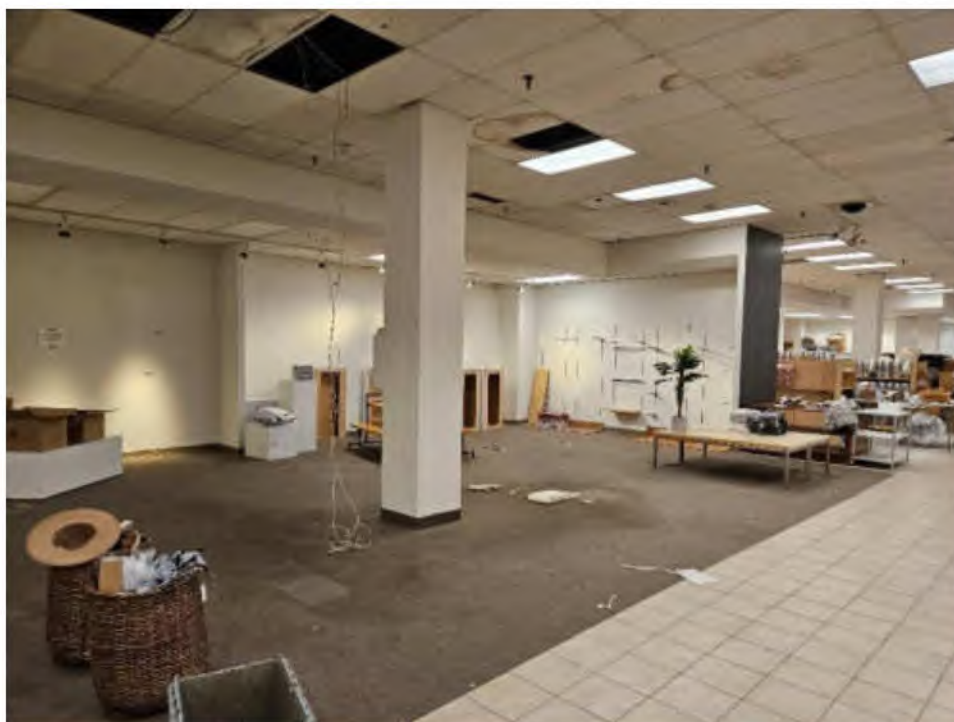
Photo #8: Example of Water Damaged Ceiling Tiles and Stained Carpet at Second Floor
