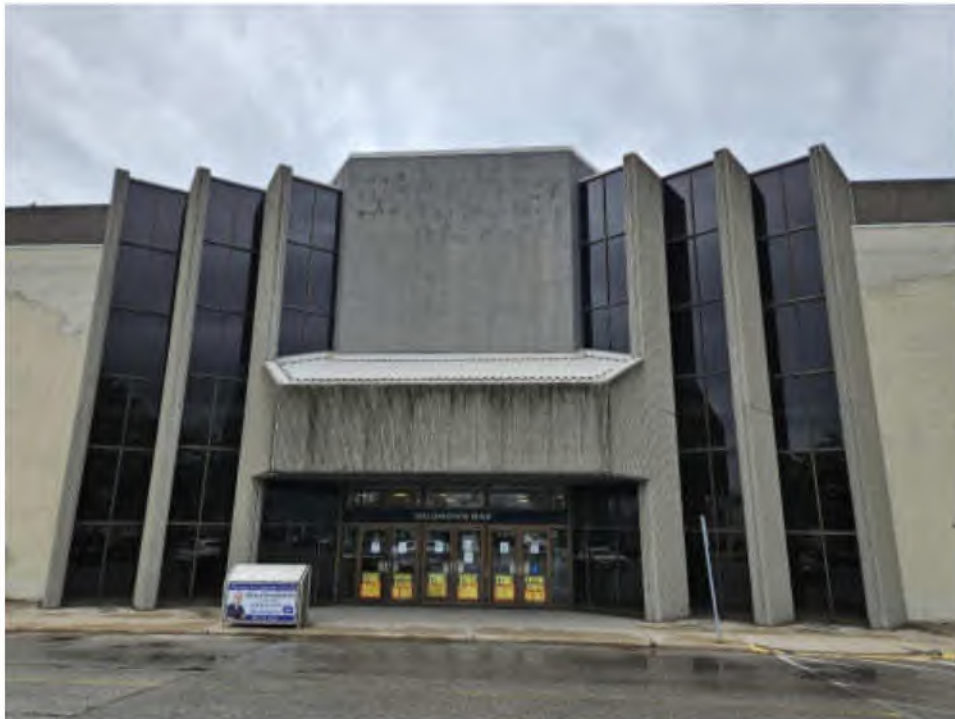
Photo #6: Typical Building Entrance (East). Note Precast Wing Walls, EIFS, and Glazed Assemblies
