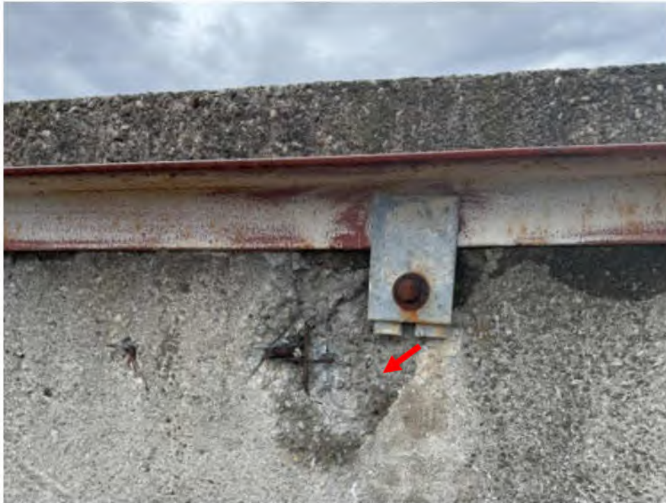
Photo #29: Localized Precast Screen Spall at Roof Side
