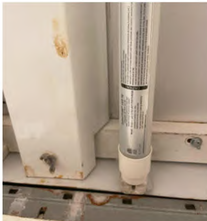
Photo #8: Retrofitted T8 bulbs inside old housing
