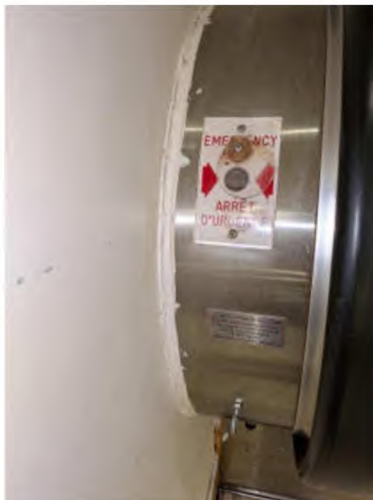
Photo #12: Escalators Emergency Controls
