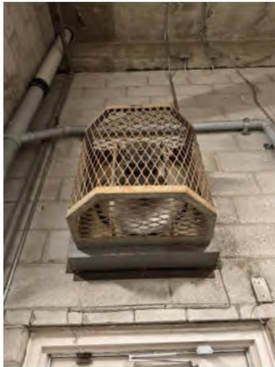
Photo #28: Garbage Room Wall-mounted Exhaust Fan
