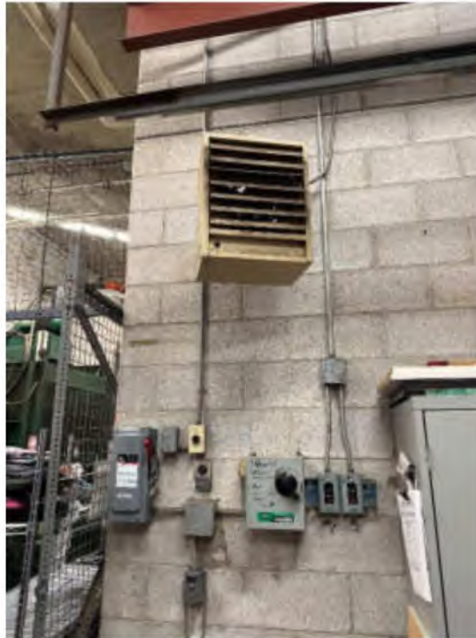
Photo #27: Loading Dock Electric Unit Heater
