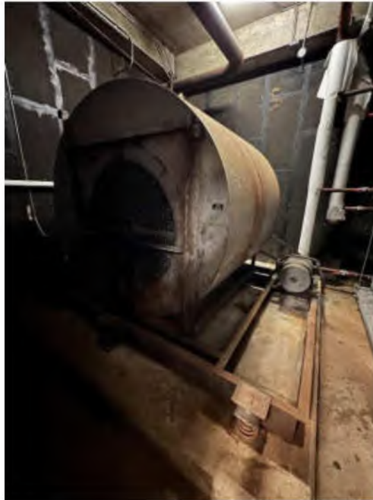
Photo #17: AHU-2 Supply Fan
