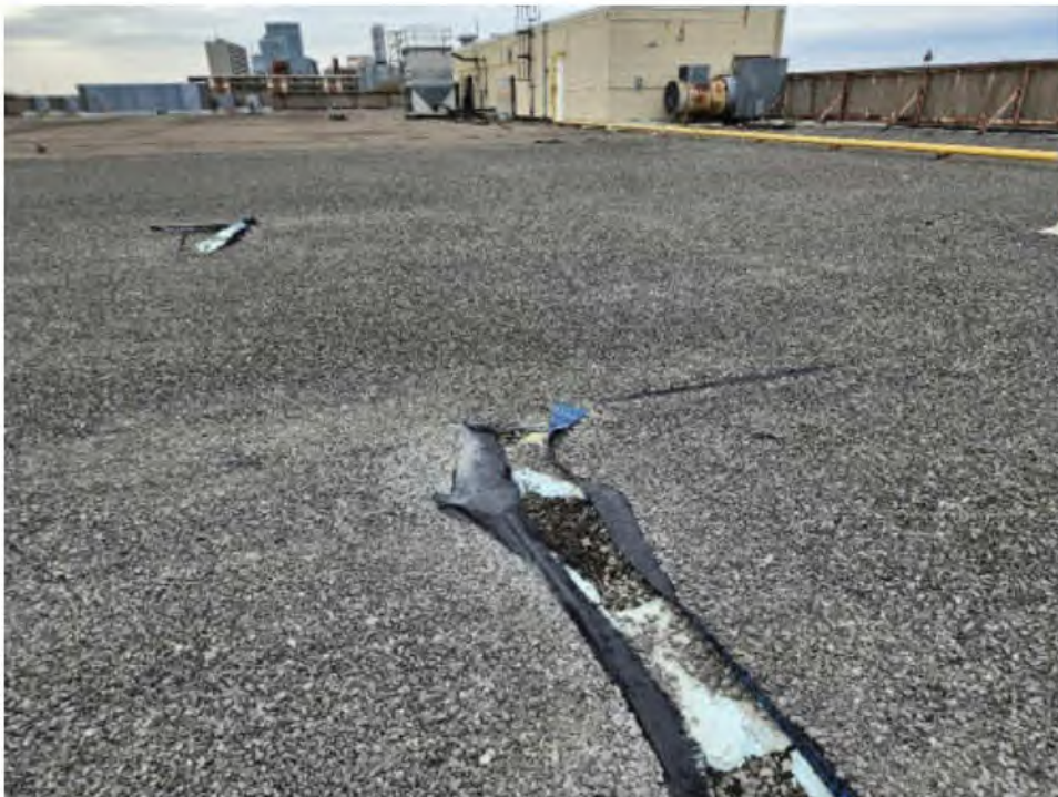
Photo #14: Example of Scoured Ballast, Torn Filter Fabric, and Exposed Insulation at IRMA Roof (Facing South)
