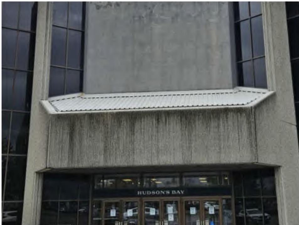
Photo #6: Typical Main Entrance Canopy with Sloped Metal Roofing and Integral Gutter
