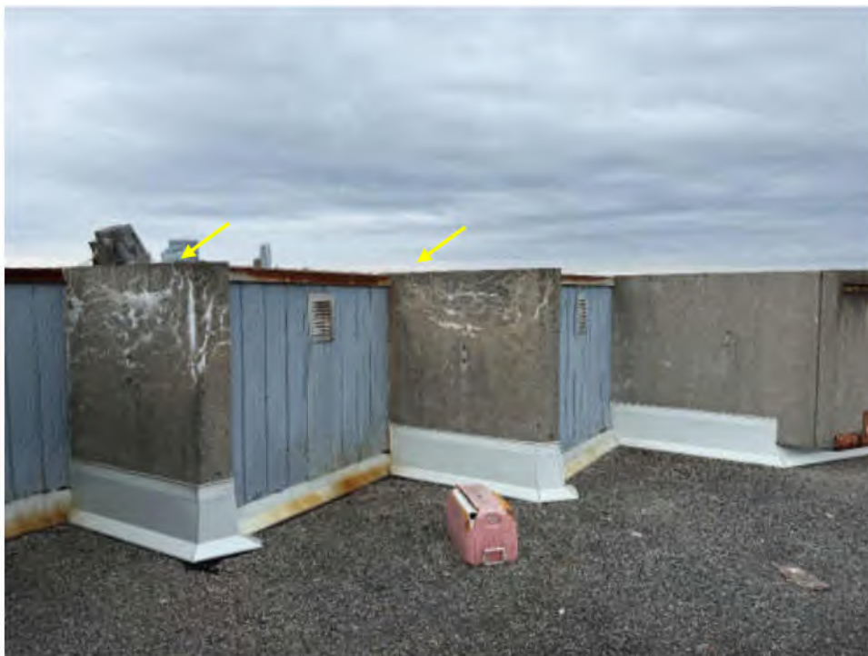
Photo #26: Localized Efflorescence at Pre-Cast Wing Wall (South End)
