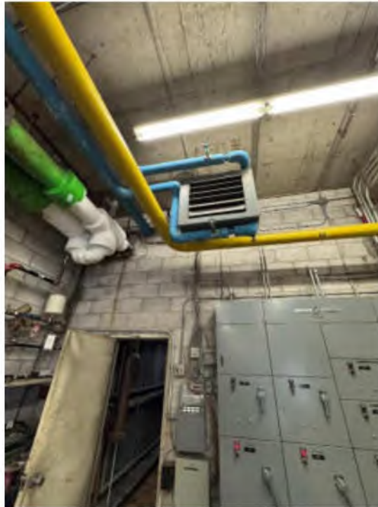
Photo #9: Mechanical Room Hydronic Unit Heater
