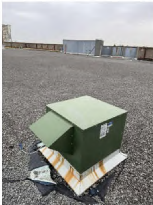
Photo #20: Rooftop Washroom Exhaust Fan
