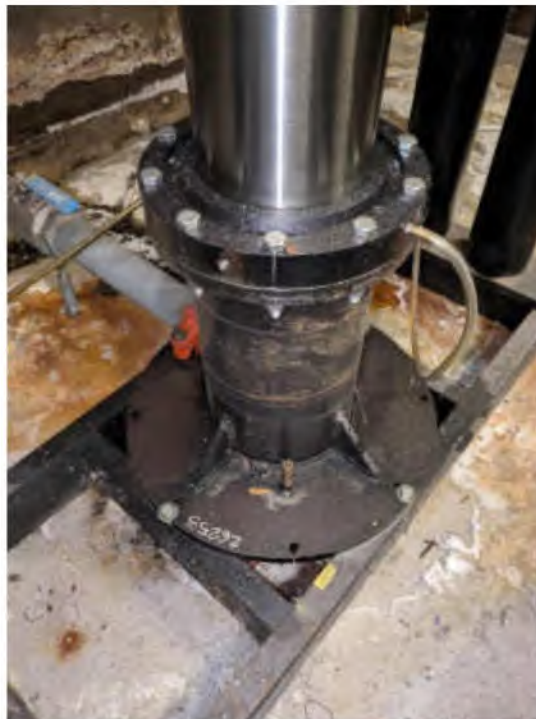
Photo #8: Freight Elevator Hydraulic Cylinder
