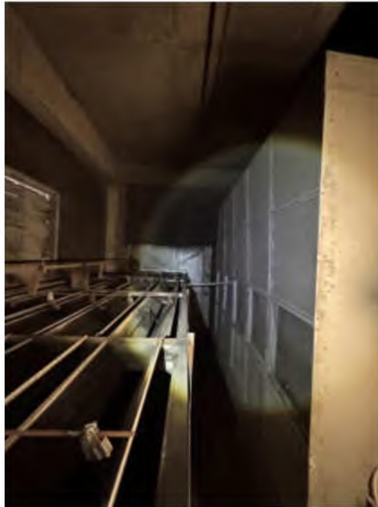
Photo #15: AHU-1 Mixing Air Plenum
