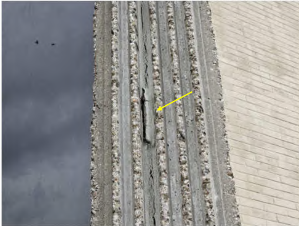
Photo #35: Example of Deteriorated Sealant Joint at Pre-Cast Wing Wall
