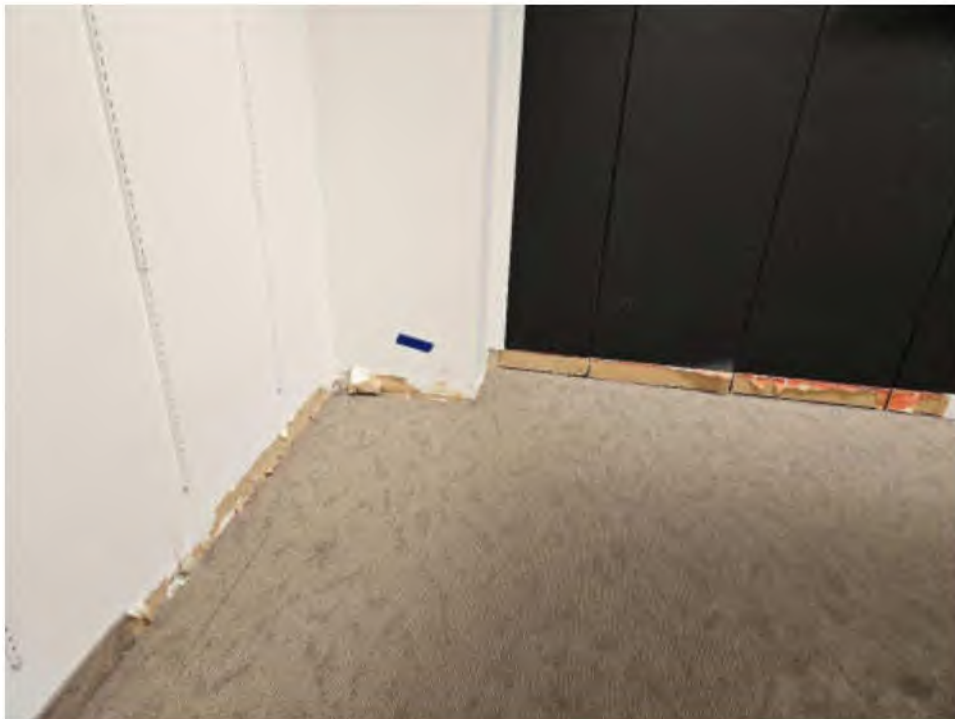
Photo #12: Example of Damaged/Missing Wall Base in Retail Space
