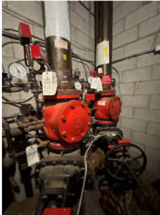
Photo #25: Main Standpipe and Sprinkler Incoming Services and Supervisory Valves
