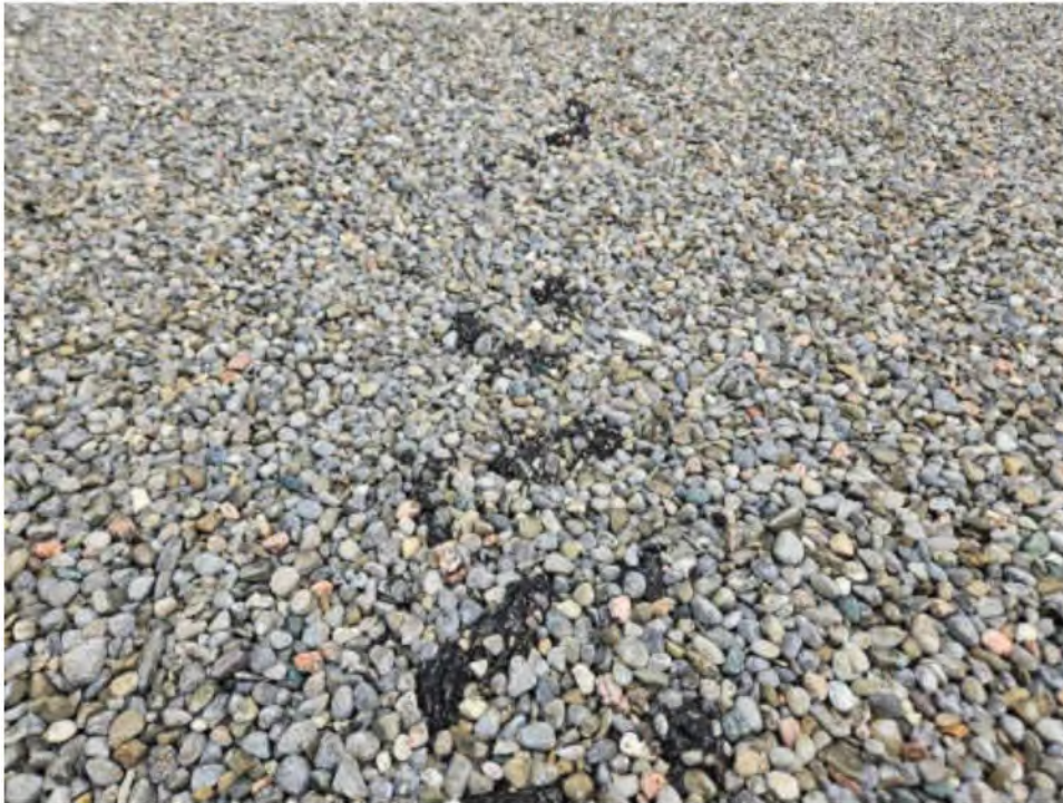
Photo #13: Asphaltic Bleed-out at Main BUR Roof
