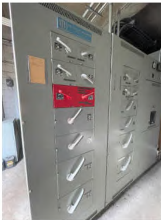
Photo #2: Main electrical switchboard
