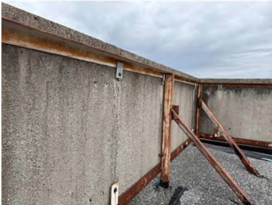
Photo #27: Typical Corrosion at Structural Framing for Roof Level Precast Screen. Potential Section Loss at Roof Pitch Pocket Flashing Detail
