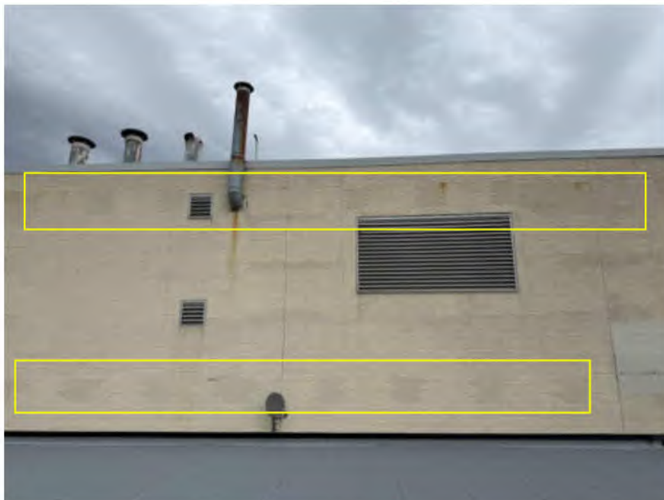
Photo #18: Overview of West Elevation, Repeating Brick Repair Pattern
