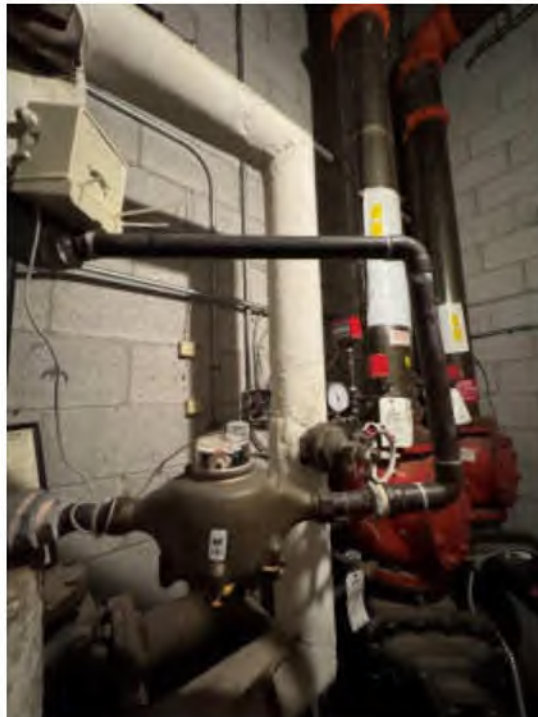
Photo #24: Main Incoming Water Service and Water Meter
