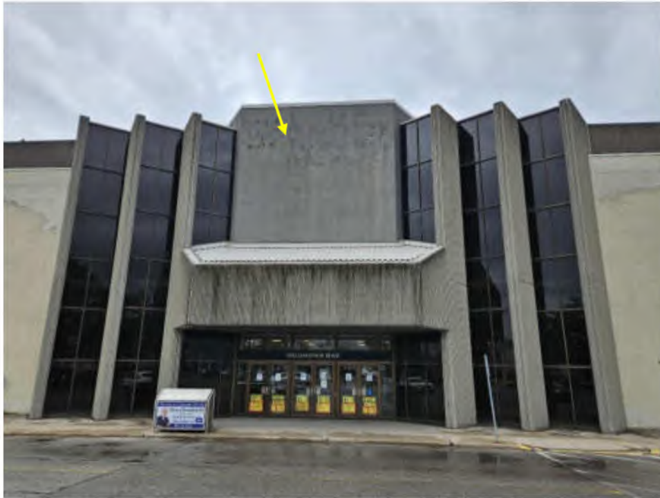
Photo #23: EIFS Installed Outboard of Stone Aggregate Wall at Main Entrances
