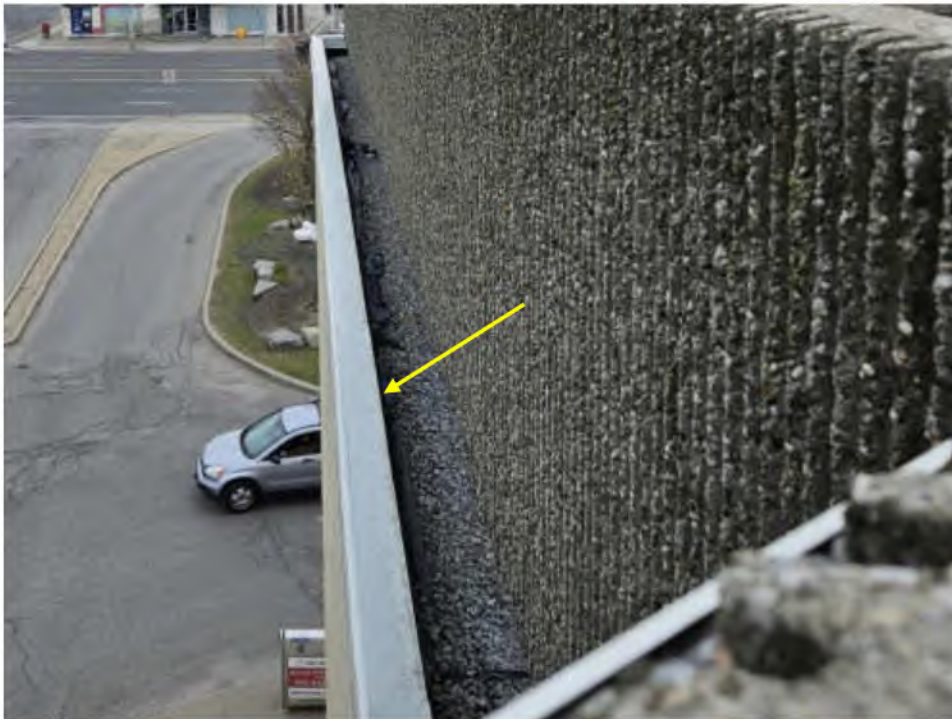
Photo #10: Typical Parapet Cap Flashing
