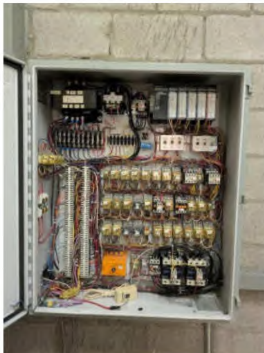
Photo #4: Passenger Elevator Controller
