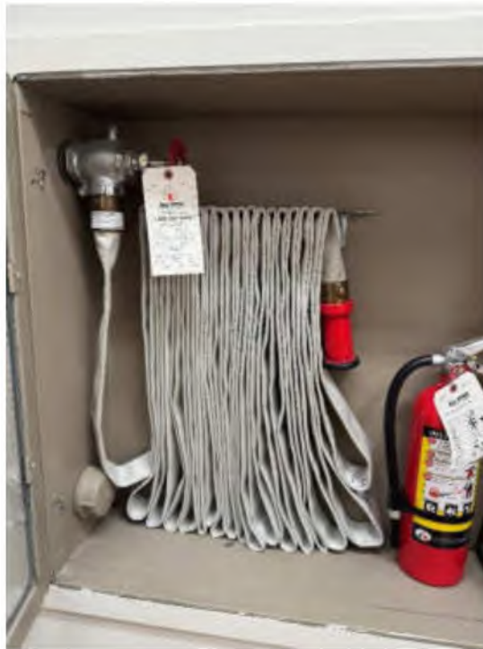
Photo #35: Typical Fire Hose Cabinet
