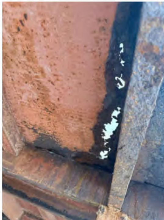
Photo #8: Underside of Steel Loading Dock (Note: Through corroded underside checker plate)
