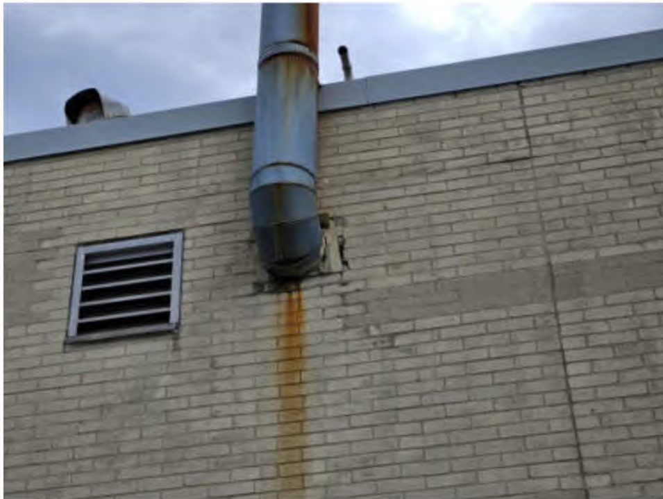
Photo #36: Damaged Brick and Unsealed Penetration
