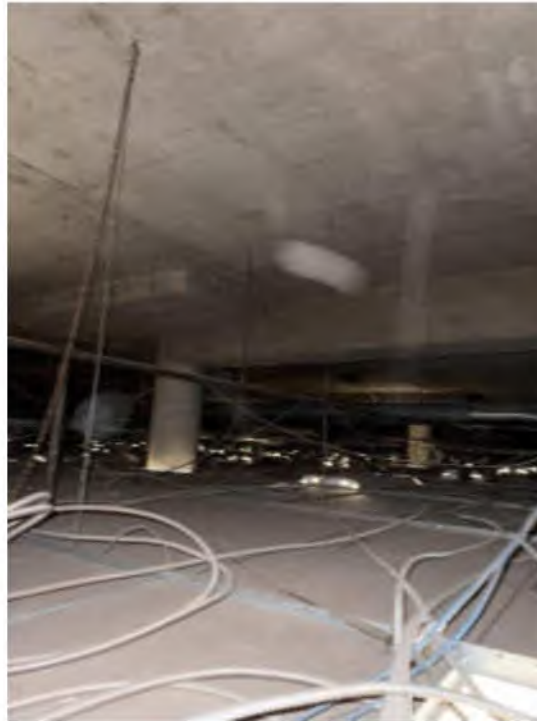
Photo #3: Underside 2 nd Floor Slab Drop Panel Augmented with Concrete Beam at South Exterior Entrance.
