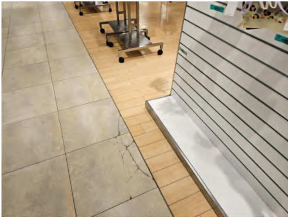
Photo #10: Example of Cracked Tile Flooring
