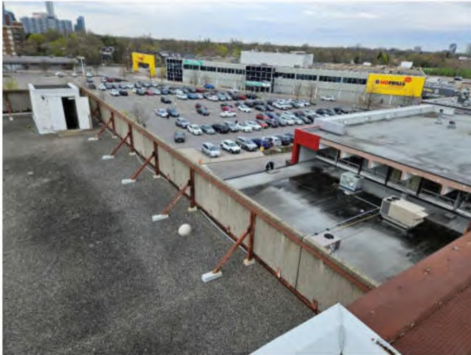
Photo #7: Typical Precast Concrete Screen at Roof Level
