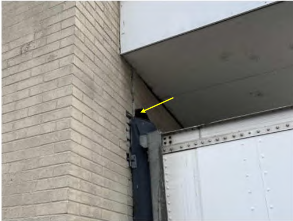
Photo #21: Brick Damaged Due to Impact Damage at Loading Bay
