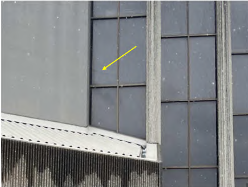
Photo #33: Cracked Glazing
