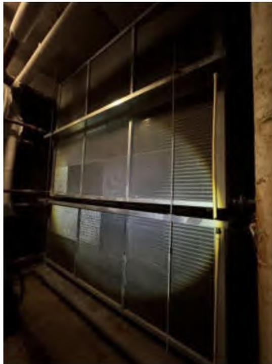
Photo #18: AHU-2 Dual Temperature Heating/Cooling Coil
