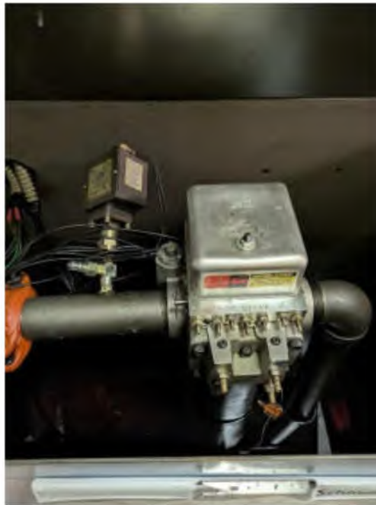
Photo #3: Passenger Elevator Control Valve
