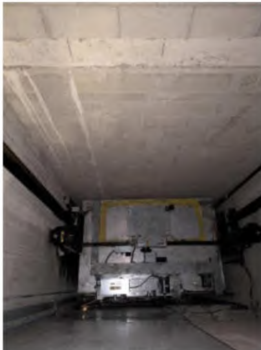
Photo #2: Passenger Elevator Car Top
