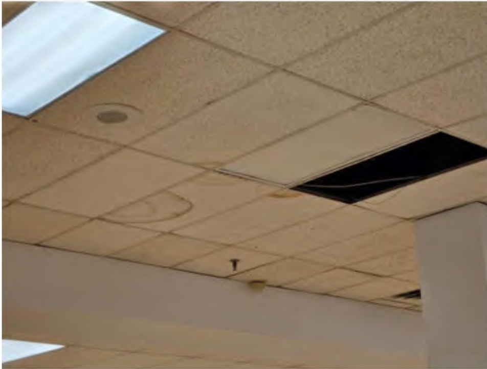
Photo #15: Stained/Deteriorated Ceiling Tiles at 2nd Floor Interior
