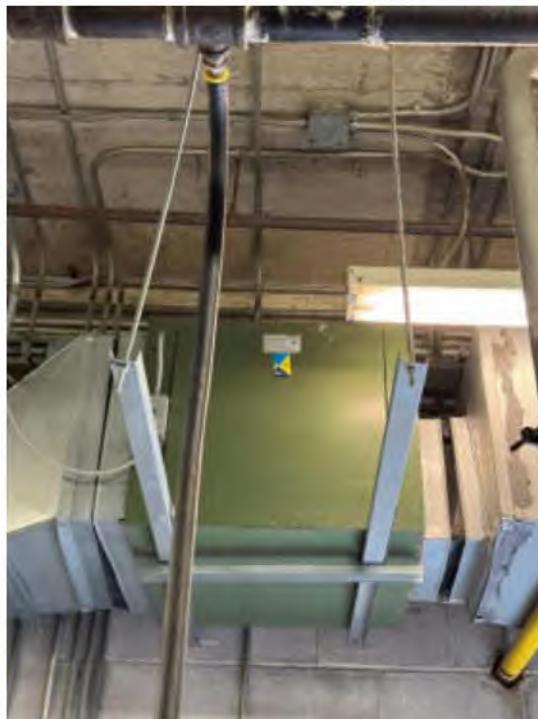
Photo #8: Combustion Air Intake Fan
