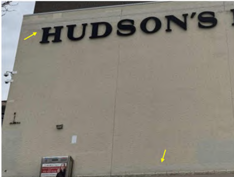
Photo #17: Typical Band Pattern of Previously Replaced Brick and Weep Holes at Ground and Roof Level
