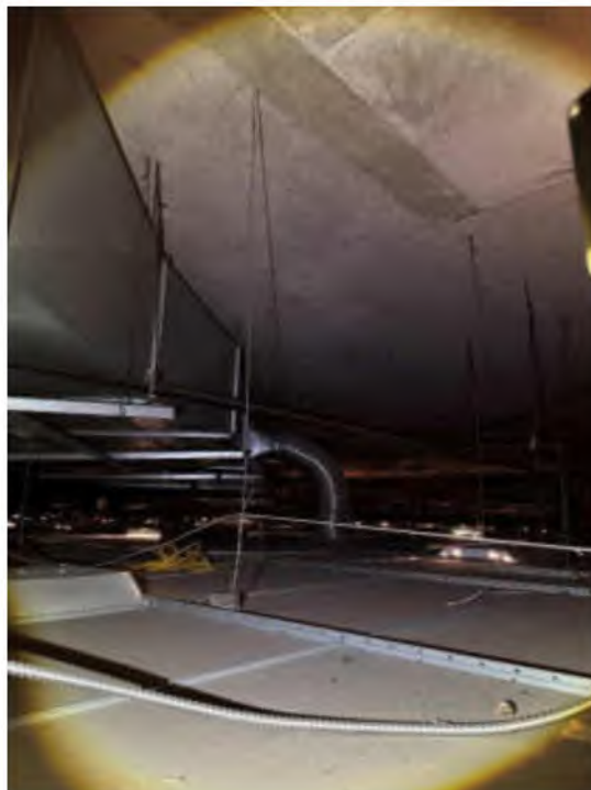
Photo #38: Above Ceiling Return Air Plenum
