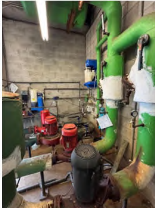
Photo #5: Chilled Water Pumps and Condenser Water Pumps
