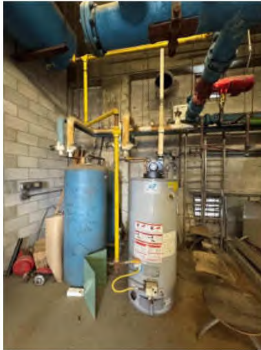
Photo #11: Gas Fired Domestic Hot Water Heater and DHW Tanks
