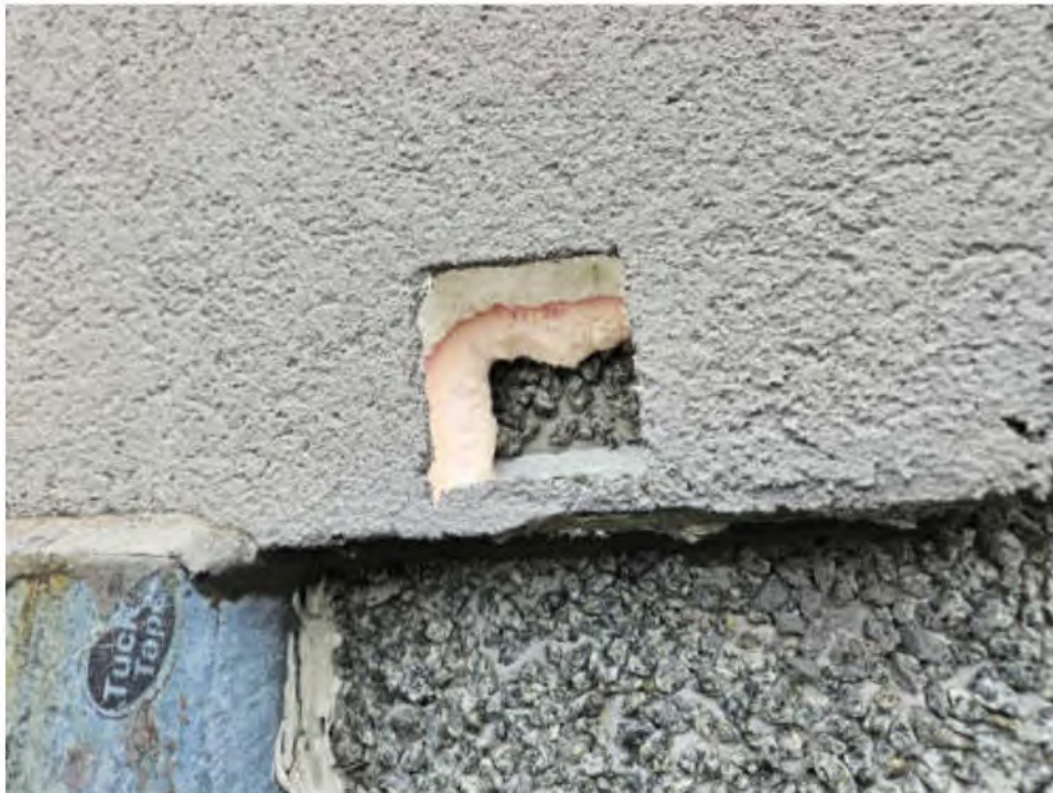
Photo #24: EIFS Overclad Existing Assembly Over Existing Aggregate on Asbestos Board
