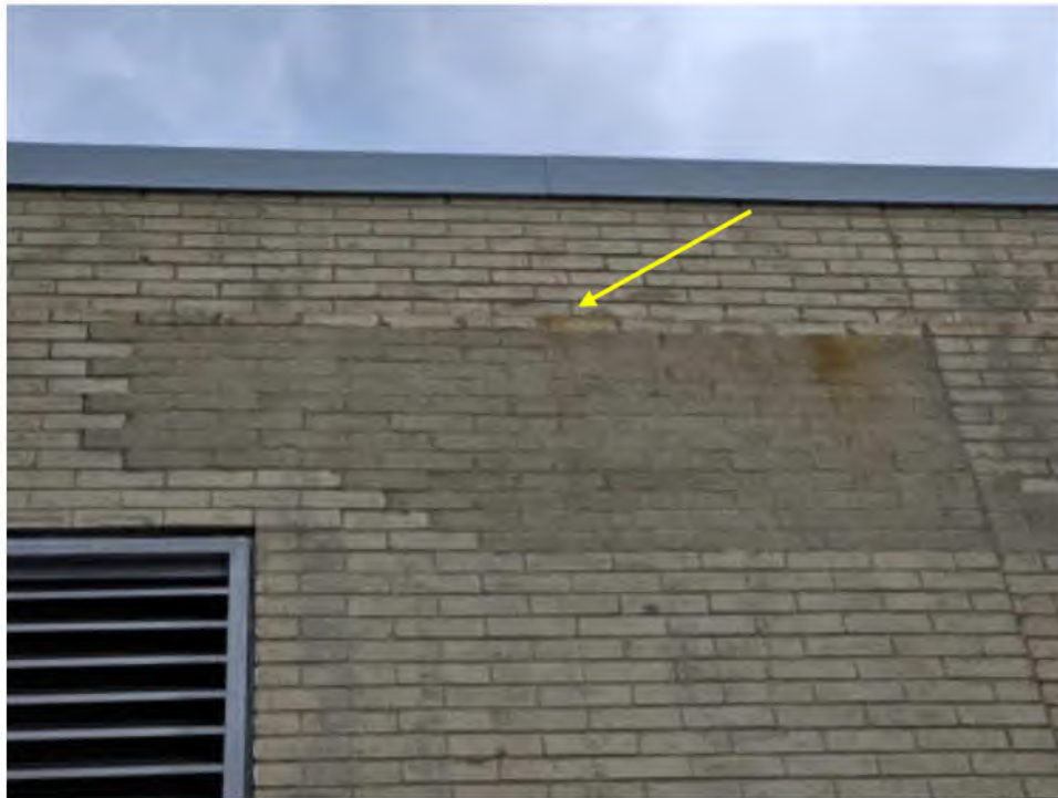
Photo #16: Section of Bricks Out of Plane at the West Elevation
