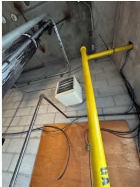
Photo #2: Generator Room Electric Unit Heater
