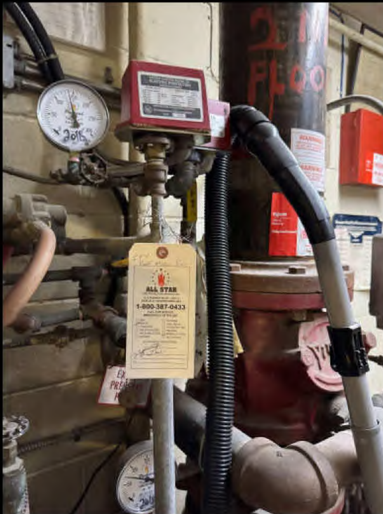
Fire Safety Systems - Main incoming water valve is in poor corroded condition
