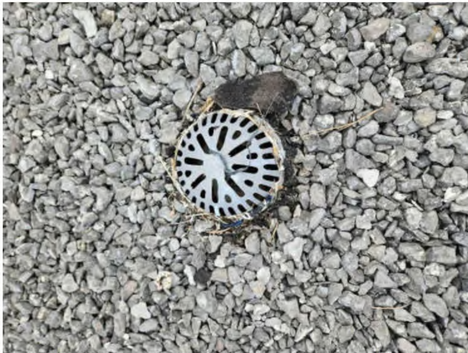
Photo #8: Typical Roof Area Drain
