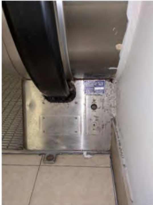
Photo #13: Escalators Handrail Inlet
