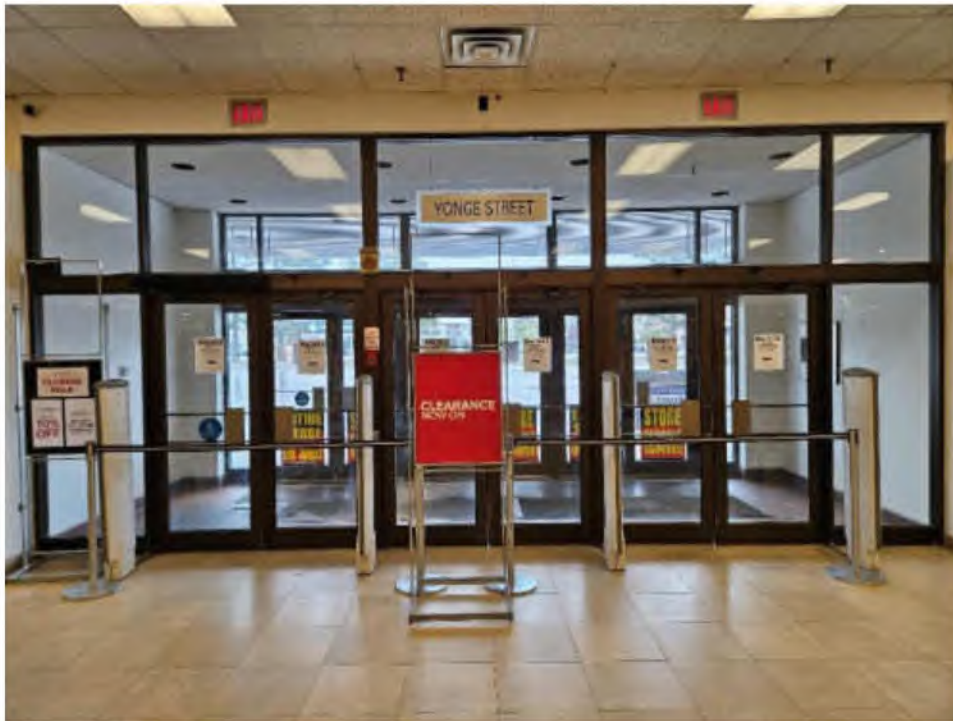
Photo #5: Typical Single Glazed Vestibule Interior Partition
