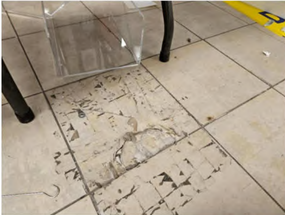
Photo #9: Example of Cracked Tile Flooring
