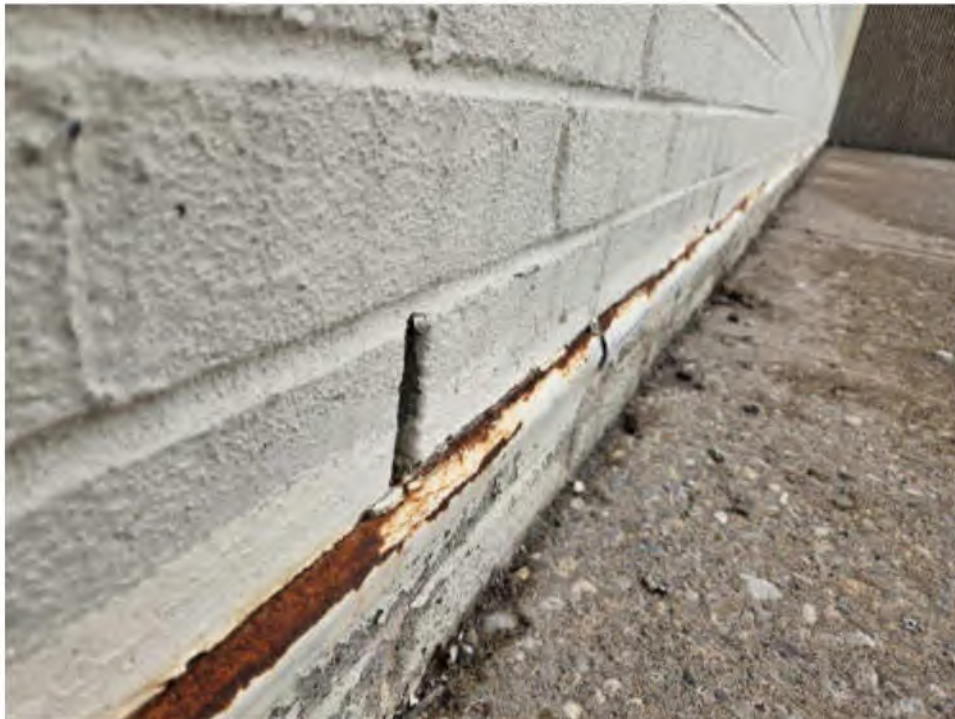
Photo #22: Typical Corroded Metal Drip Edge Flashing
