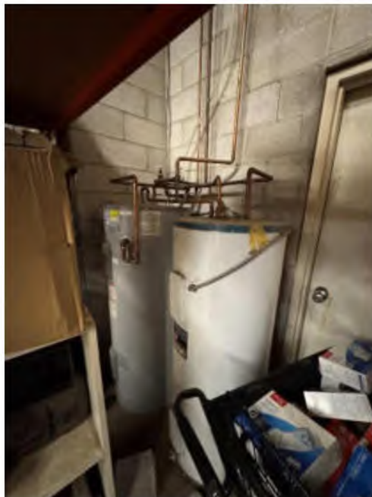
Photo #22: Electric Domestic Hot Water Heaters
