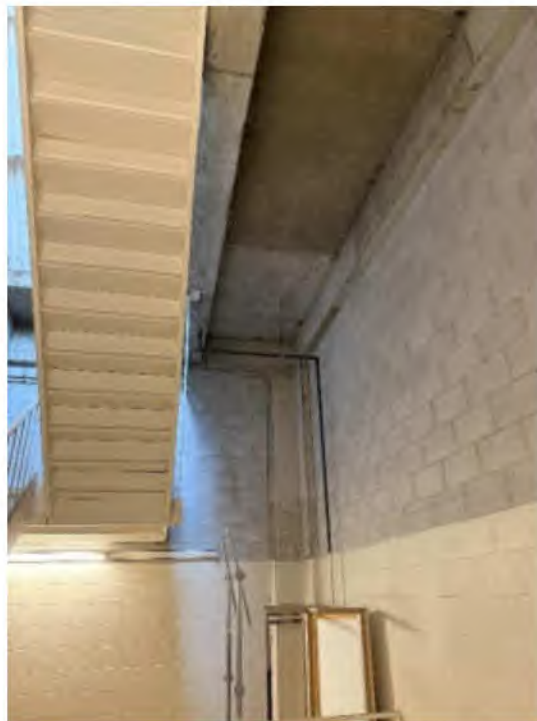
Photo #4: Southwest Stair Well. Concrete Structure with Metal Staircase
