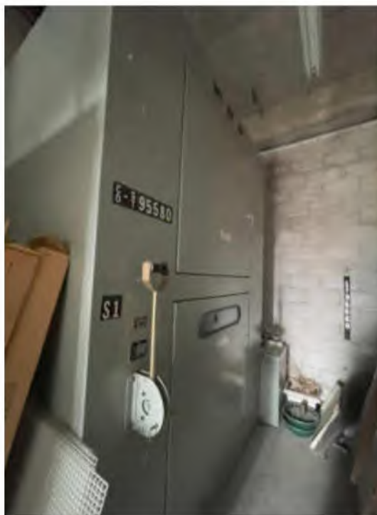
Photo #1: Main HV switch
