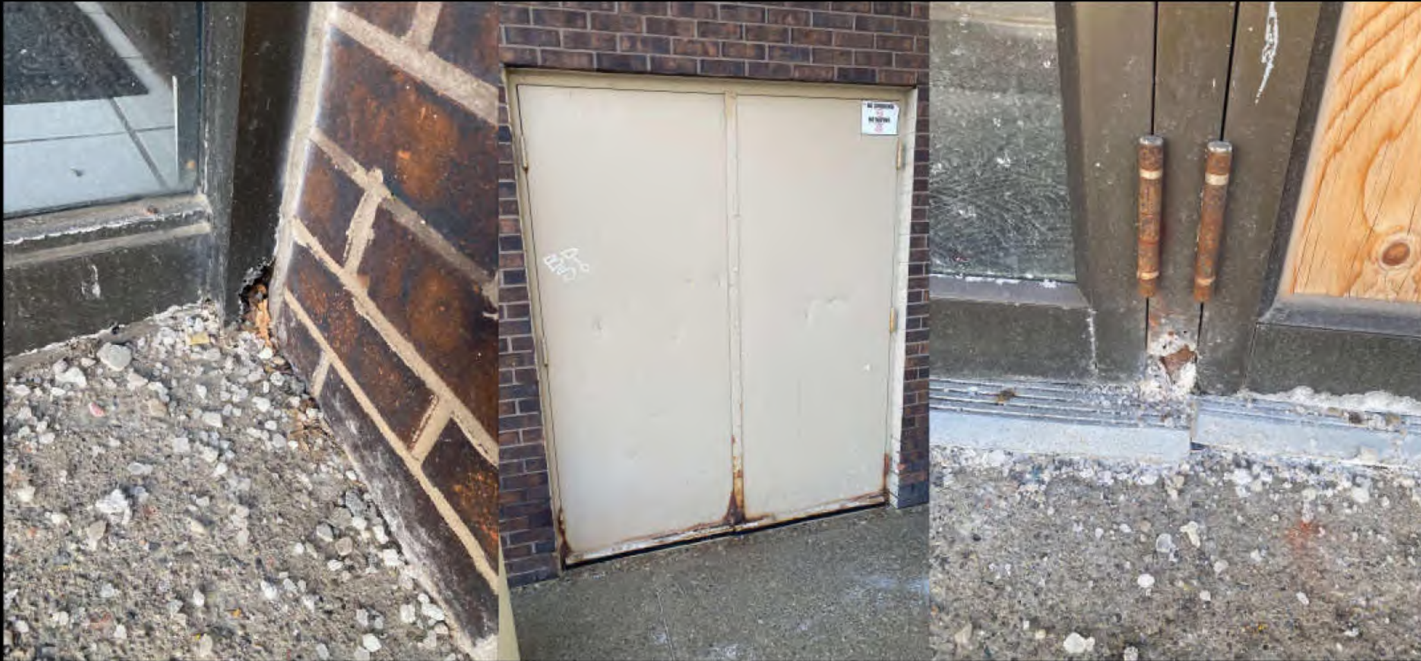
Exterior - Corrosions/Damages to Entrance and Egress doors
