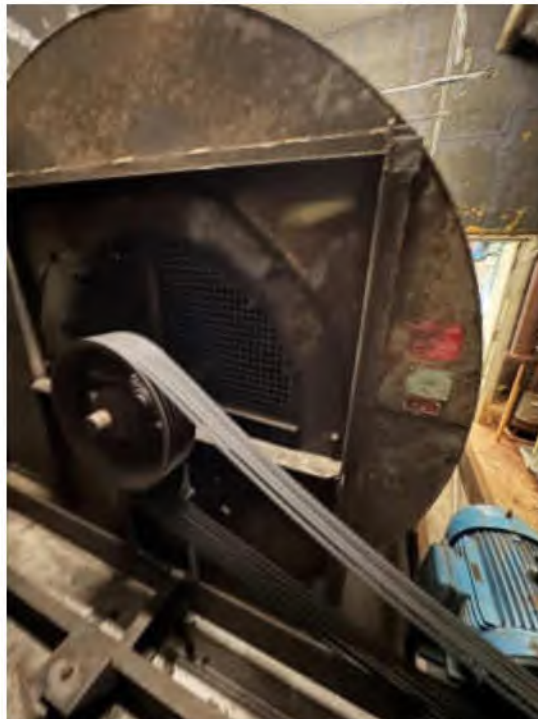
Photo #14: AHU-1 Supply Fan Belt Drive Motor
