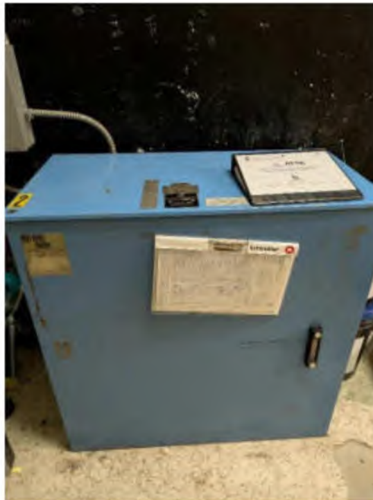
Photo #5: Passenger Elevator Power Unit and Tank
