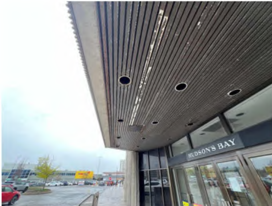
Photo #7: Typical Metal Soffit at Entrance
