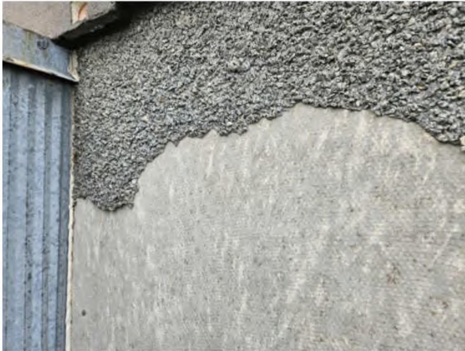
Photo #25: Delaminating Stone Aggregate at Roof Level Exposing Underlying Asbestos Board Substrate
