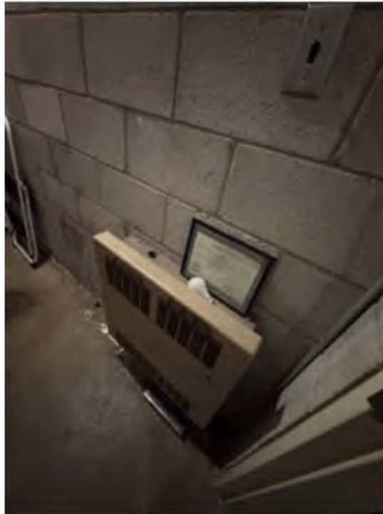
Photo #23: Sprinkler Room Forced Flow Heater
