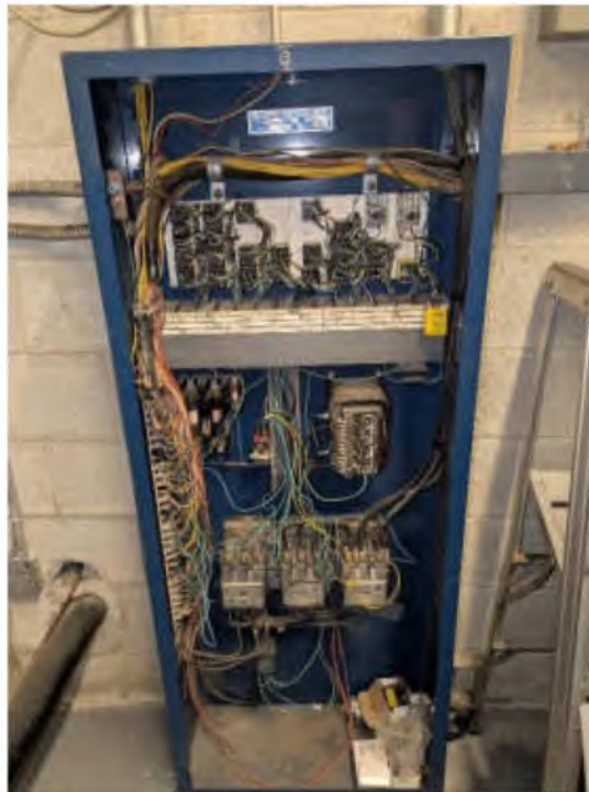
Photo #7: Freight Elevator Controller
