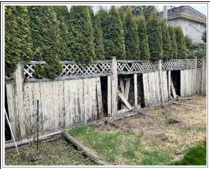
CRACKS OF FENCE AT REAR
