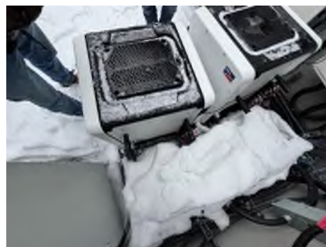
Figure 6-3 Mounting of inverters
