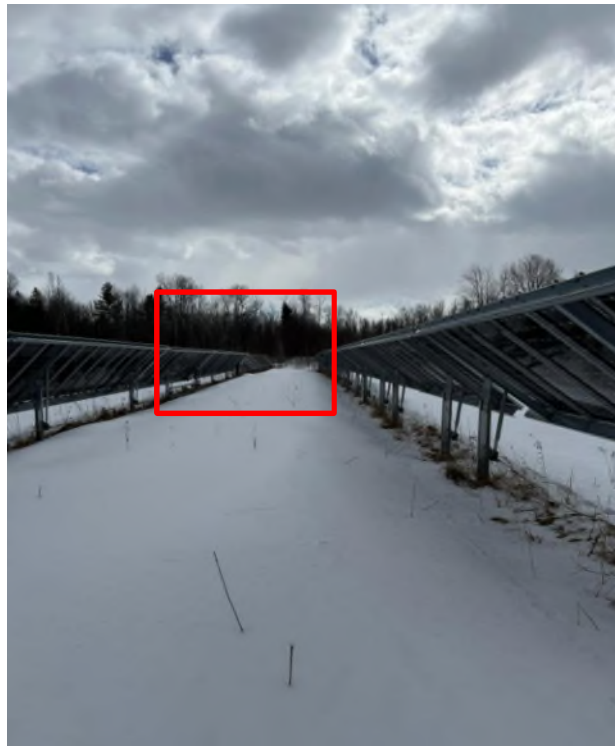
Figure 6-6 Modules facing different directions within the same row
