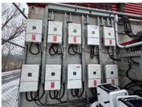
Figure 6-3 Mounting of inverters
