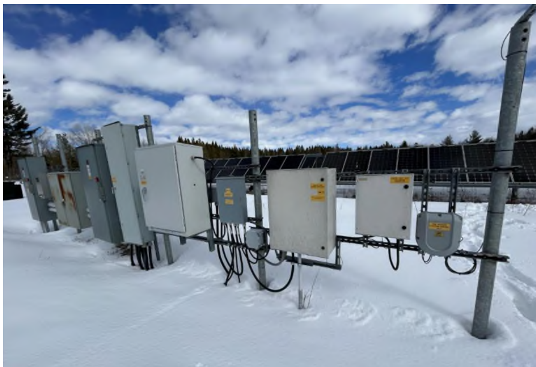
Figure 6-12 AC collection system
