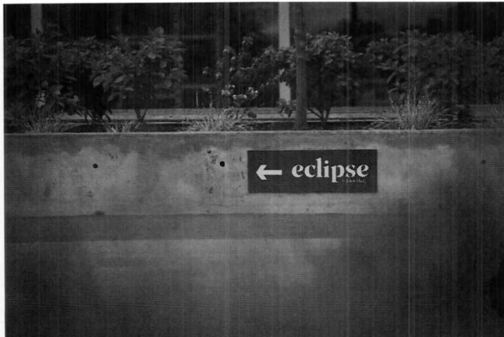
Construction at the Eclipse condo tower was 'deemed substantially complete' by mid-March, but more than three dozen pre-sale purchasers are asking a B.C. Supreme Court judge to declare their contracts unenforceable. (Nav Rahi/CBC)
