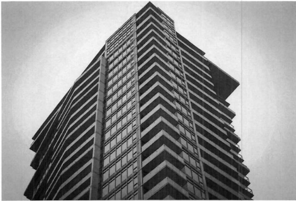
Burnaby's Eclipse condo project was placed into creditor protection in January 2025. The 34-storey development was 95 per cent complete at the time and 232 of the tower's 329 units were sold. A number of pre-sale purchasers have accused the developer of breaching B.C.'s Real Estate Development Marketing Act. (Nav Rahi/CBC)
