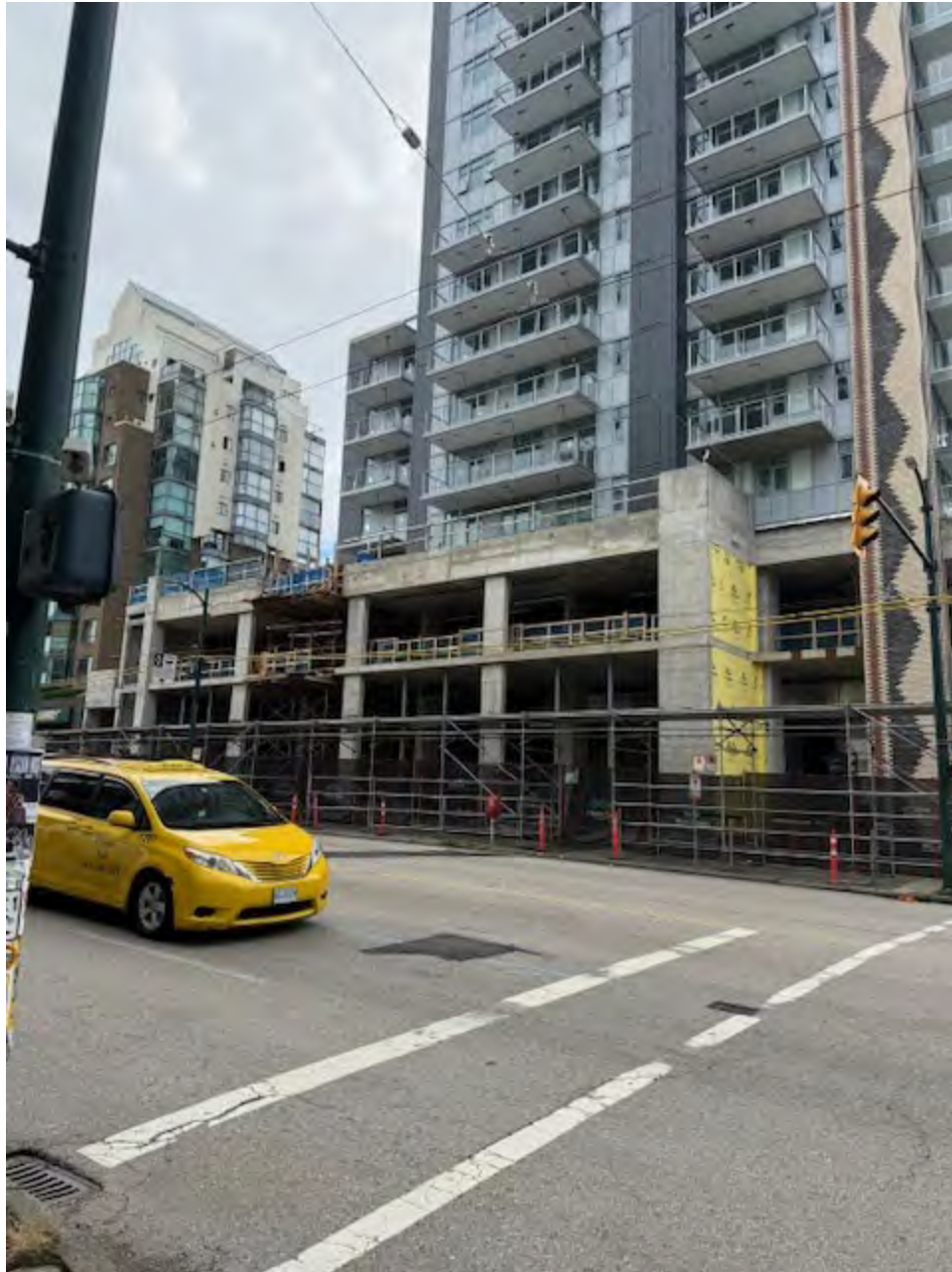
Subject Photo 6 View of commercial levels along Broadway
