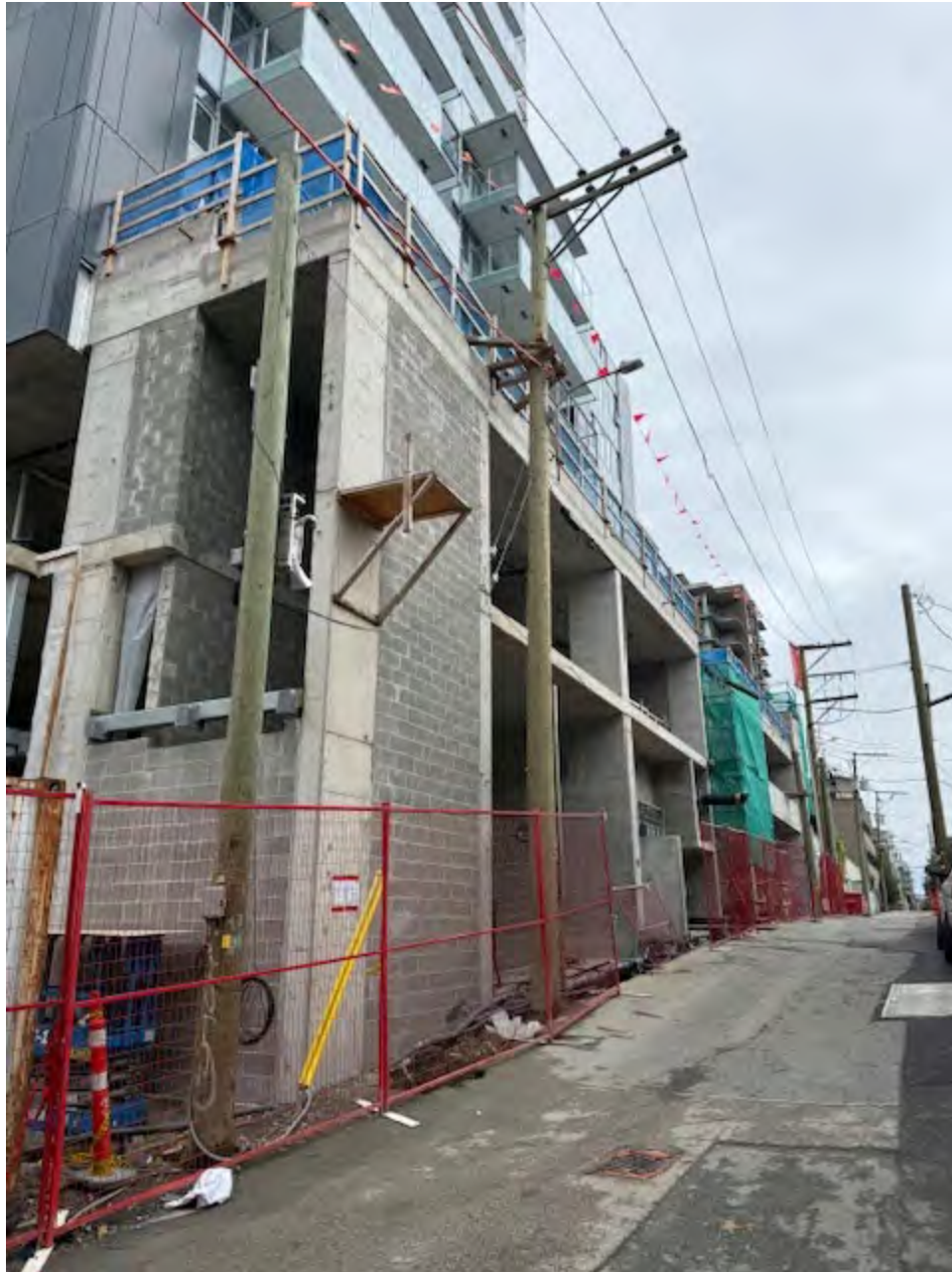
Subject Photo 5 View of rear lane.
