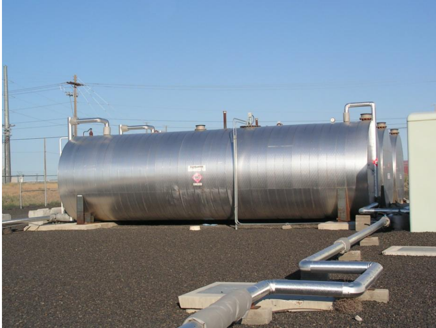
20,000 Gallon Fuel Tank Setup
