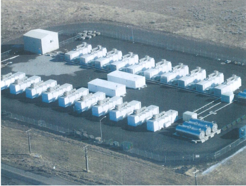
Gensets - Moses Lake Public Utility Configuration – (eight of the above units are being offered for sale by the Receiver)
